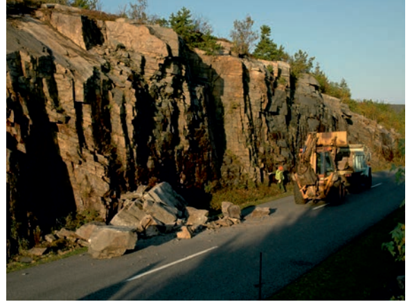
Şekil 8.1. Kaya düşmesisonucunda zarar gören yapılara bazı örnekler ( http://www.nps.gov/acad/photosmultimedia/Earthquake-Effects.htm ; http://blogs.agu.org/landslideblog/2011/02/23/on-the-causes-of-the-high-levels-of-loss-in-the-christchurch-earthquake ).
