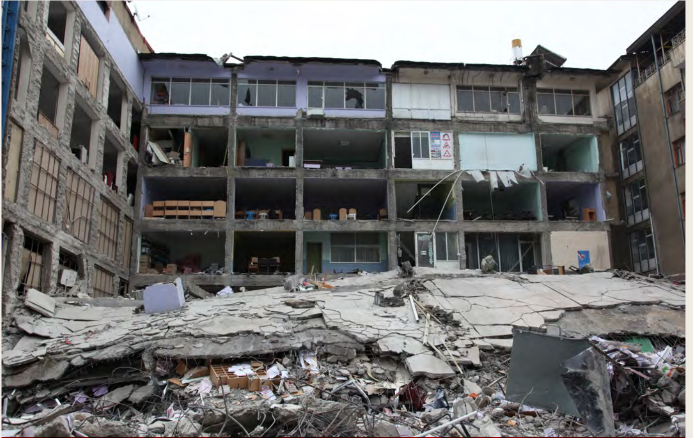
2011 Van Depreminde Tamamen Yıkılan Otelin Enkazı - Ruined Hotel Wreck in 2011 Van Earthquake
