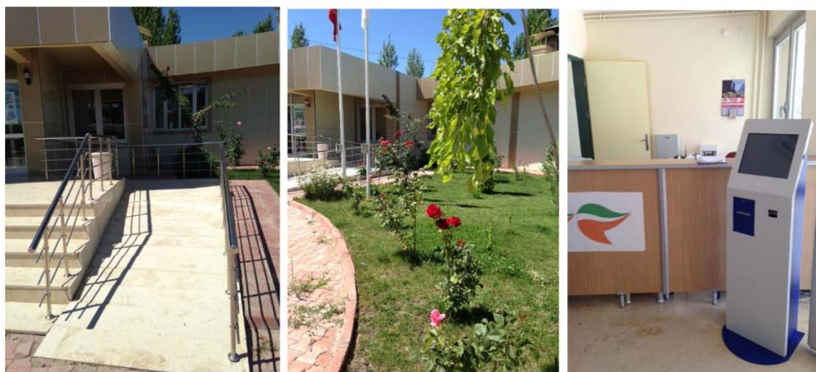
Fig. 8. Rural Family Medicine Centre in Malatya Province with a disabled ramp and queuing system
